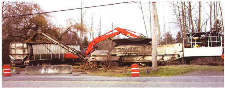
Mulching and recycling vegetation with a big tub grinder
